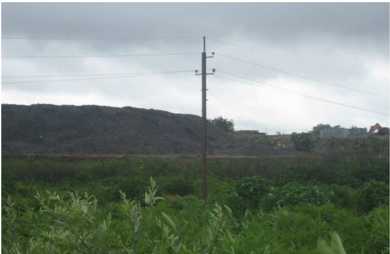
Figure 7: A view on CMSK installation at LUSWICHI
